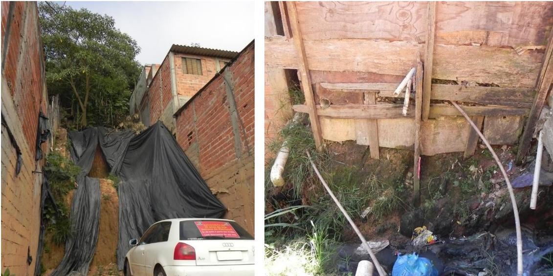
On the left photo, two vertical cuts were made, and soil was protected with a plastic cover observed in Jardim Brilha neighborhood (Mairiporã city). On the right photo, sanitary system absence is observed in *favela* 'Encosta do CEU Paz': wastewater is disposed of directly into a drainage channel, which also carries garbage from upper areas.
