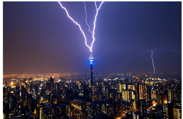
Figure 9. Photograph lightning event to Hillbrow tower taken from the Ponte building. Courtesy Jonathan Wood.
