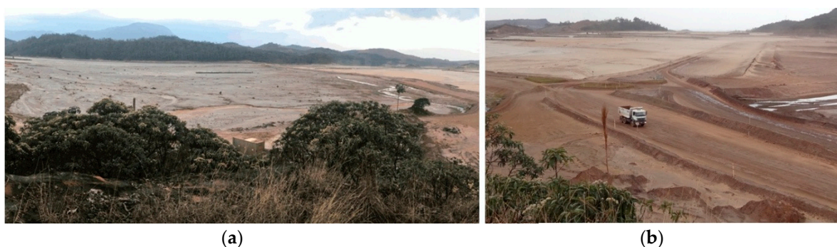
Figure 19. Field picture of the Baía 3 dam and its reservoir (a) and the auxiliary dike that cross the Germano reservoir (b).
