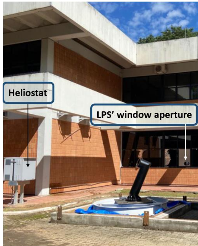
Figure 4.3 (a) shows the exterior of the LPS building with highlight the closed heliostat and the aperture of the window. (b) represents a drawing of the internal layout of the LPS. One can see the opening through which the light enters, the optical table, and the PCPS.
